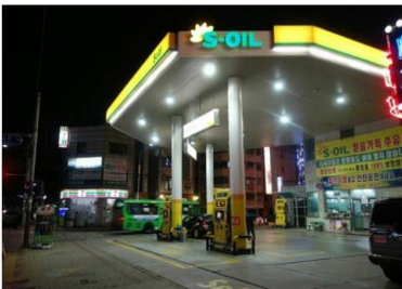
Gas station, Incheon
