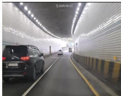
Tunnel, Ansan (Wongok)
